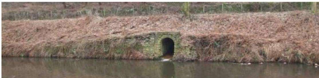
**This is where the drain water exits the underground channel and flows into the canal.**
