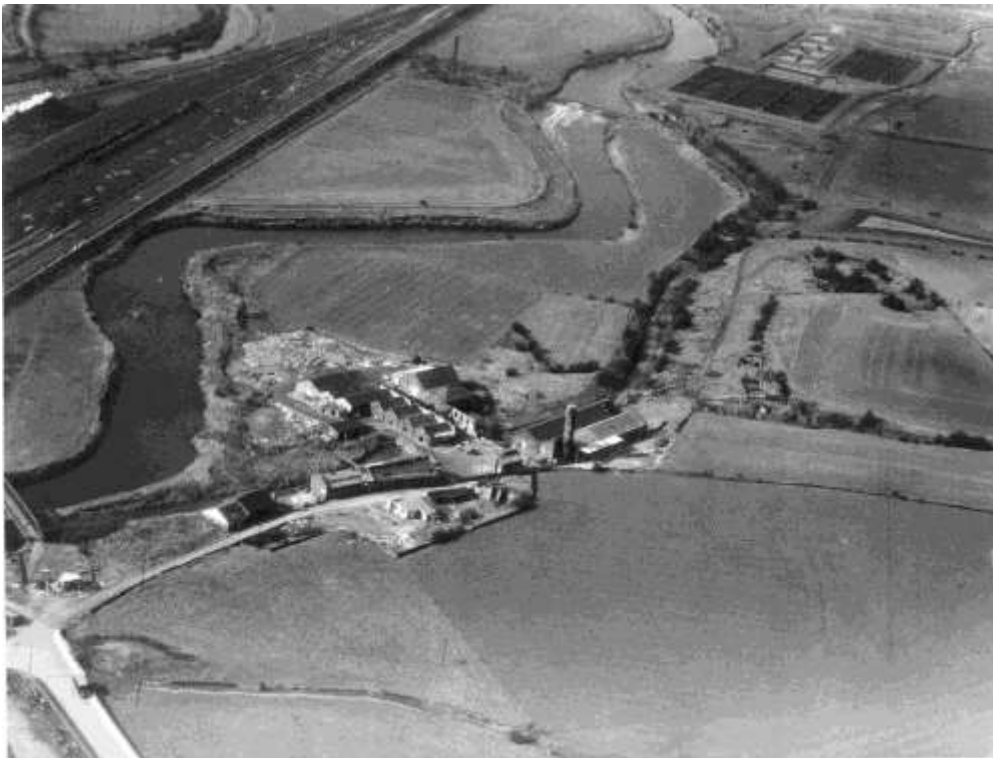
Healey Old Mill Yard post 1961. The tree lined goit or mill race which once took water from the Calder & through the Mill to power the water wheel can be clearly seen. Photo Mark Allen
